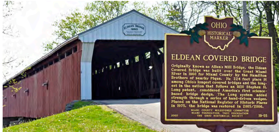
Eldean Bridge ▲ Built in 1860, Eldean Bridge is the longest “Long Truss” covered bridge in the country spanning 224 feet. Its historical significance earned it a spot on the National Register of Historic Places in 1975, and in 2016, it was further honored as a National Historic Landmark.
